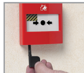
Step 3: To reset a simple key is inserted into the bottom of the call point.
